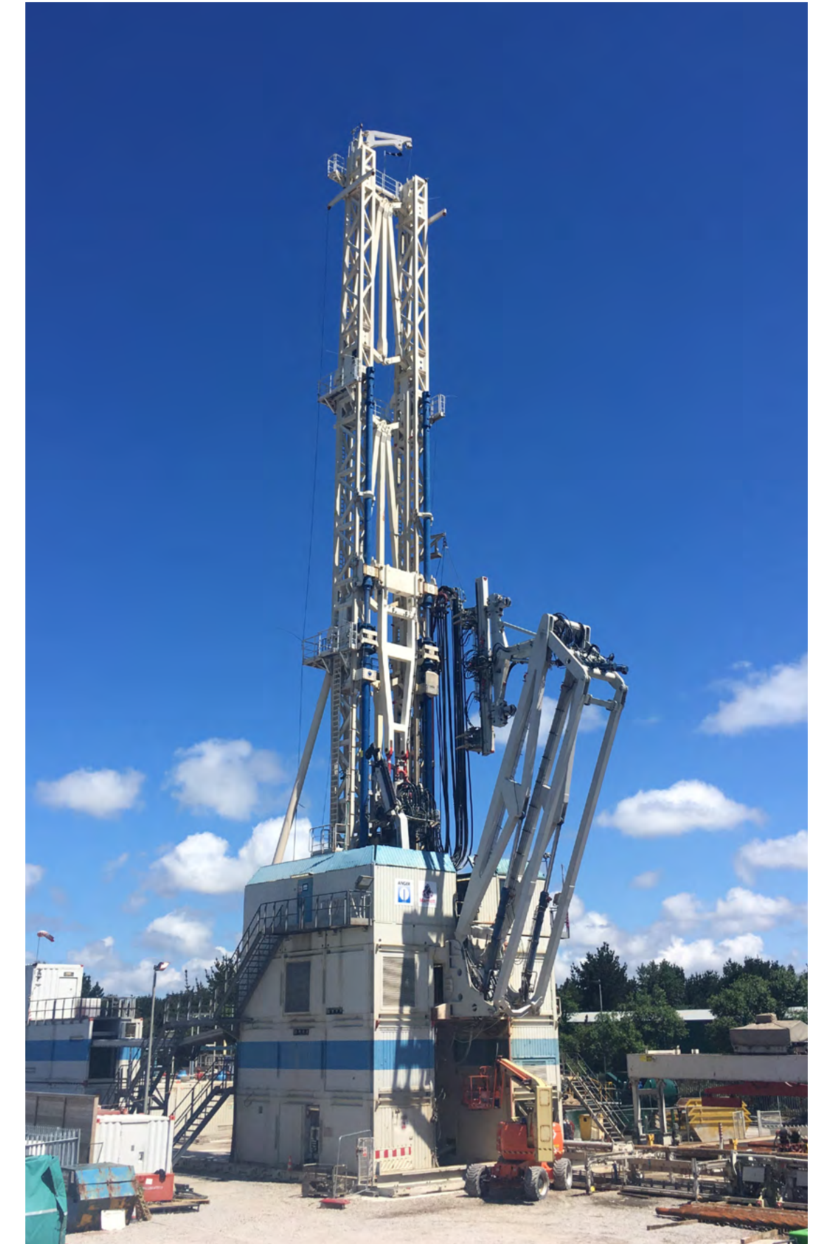
Drilling rig at the United Downs project in Cornwall © photograph courtesy of Geothermal Engineering Ltd
